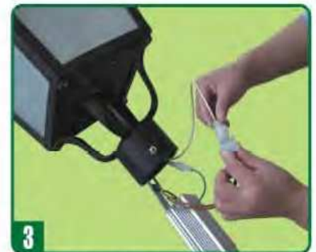
3 Connect the two-hole quick connector of the lamp wire.
